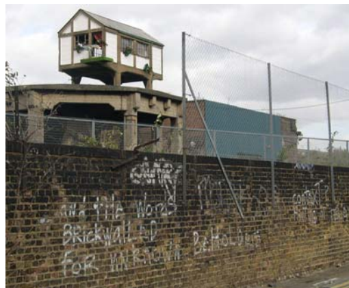
The transformation by OSA and Trent Oldfield of an old signal box above a railway in East London
