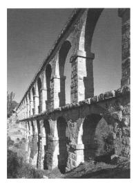
The aqueduct of les Ferreres, also known as Pont del Diable (Devil's Bridge) is located near Tarragona. It was constructed during the time of maximum apogee of Tarraco, in the 1<sup>st</sup> century A.D. The highest point reaches 23,7 m and its length is 217 m.
