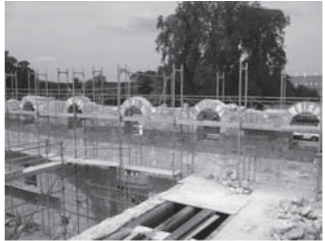
Figure 18. Stone arches for the windows of the basilica thermarum in the public bath (2010) (Franz Humer, Haslau a.d. Donau).
