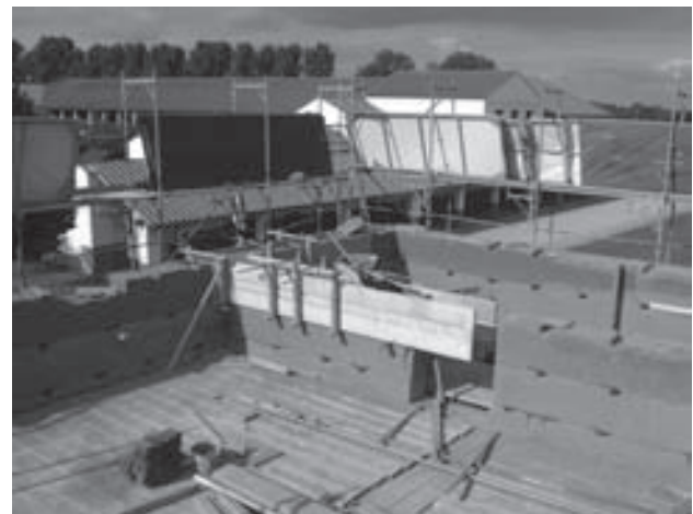
Figure 18. Xanten Archaeological Park. Rammed earth technology used to reconstruct three Roman artisan houses in experimental archaeology (P. Kienzle).
