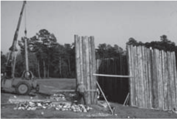
Figure 7. Reconstructing the north prison gate at Andersonville National Historic Site, Georgia (Courtesy, National Park Service).
