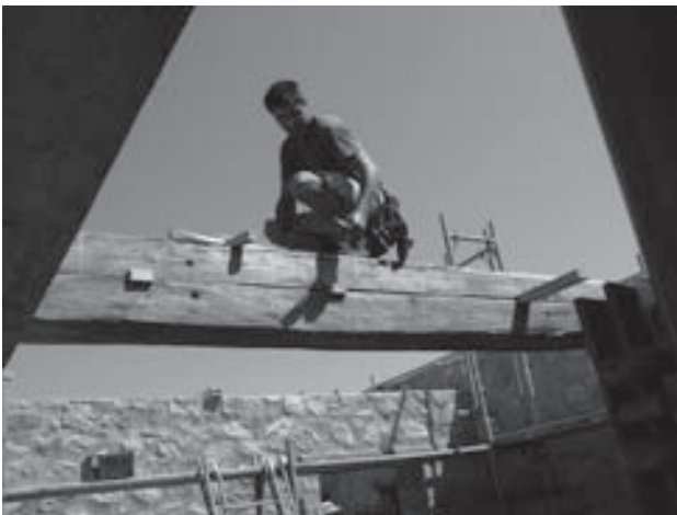
Figure 17. Using old methods of handcrafts for making the wooden constructions in the public bath (2010) (Franz Humer, Haslau a.d. Donau).
