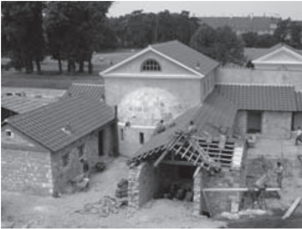
Figure 9. Work in progress reconstructing a villa urbana in situ using original materials (2008) (Franz Humer, Haslau a.d. Donau).
