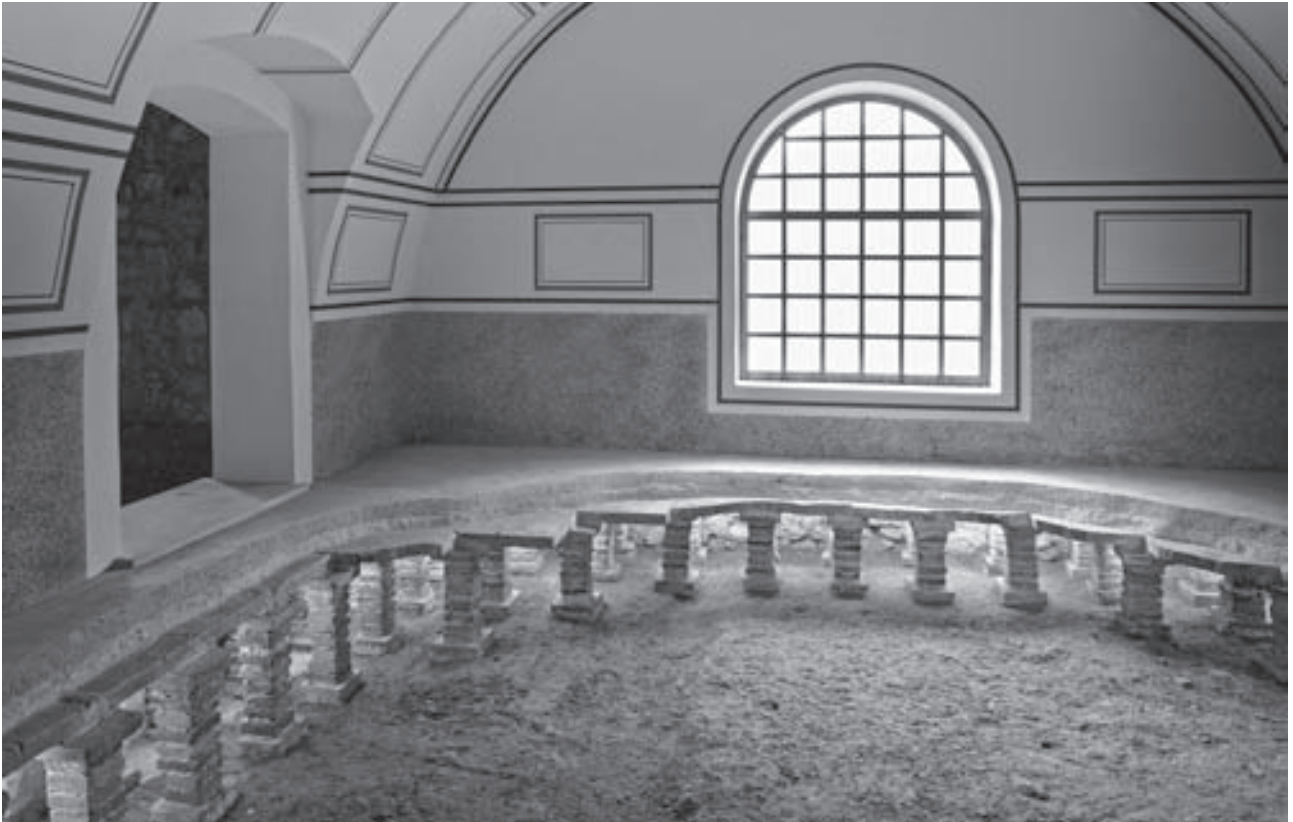
Figure 16. Reconstructed hypocaust -structures in situ above original layers from the 4 th century AD in the public bath with the reconstructed building for protection (2010) (Atelier Olschinsky, Vienna).
