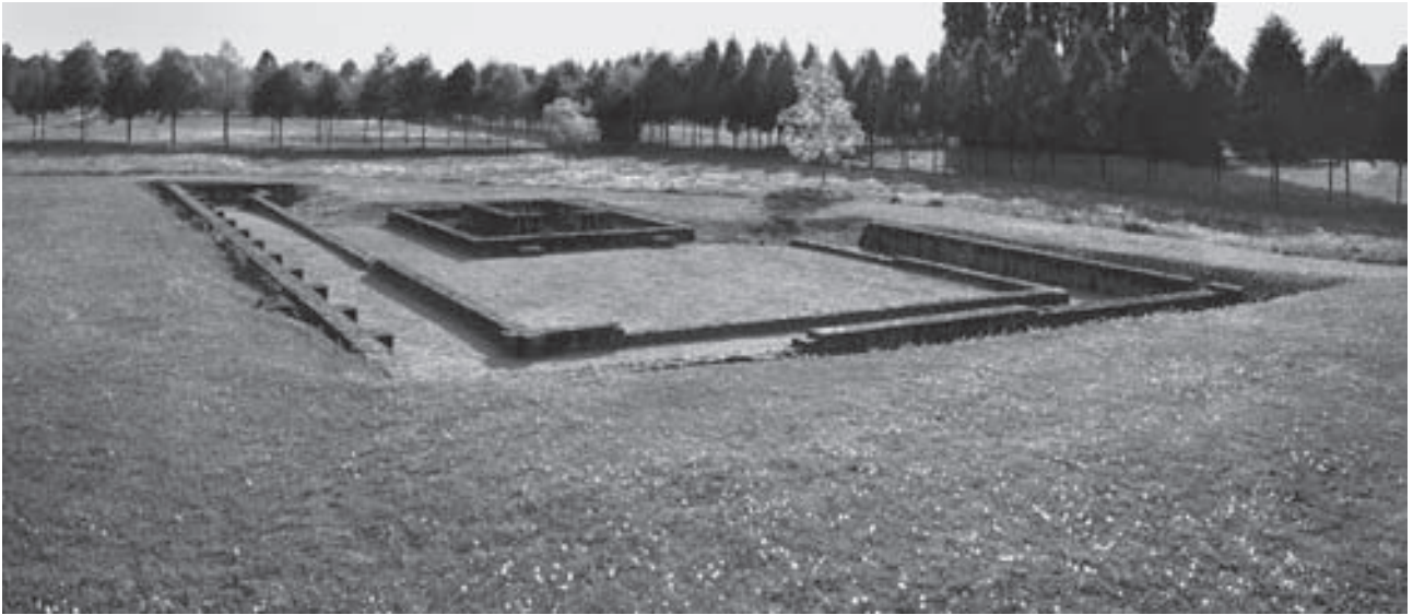
Figure 11. The exposed original foundations of a Gallo-Roman temple in the Xanten Archaeological Park were protected with capping of modern masonry (A.Thünker, DGPh).
