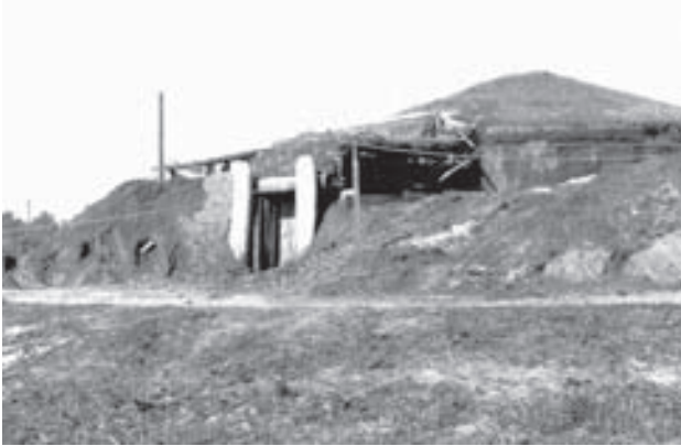
Figure 1. Photo taken during the 1930s reconstruction of a Mississippian period earth lodge, Ocmulgee National Monument, Georgia (Courtesy, National Park Service).
