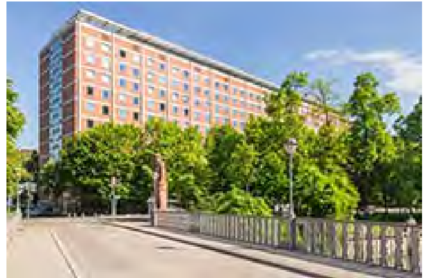
GPTO headquarters in Munich
